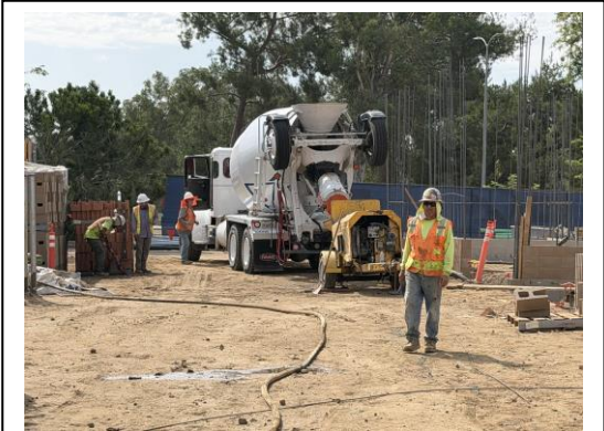
Construction progress on the Plant Facilities Warehouse and Shop at Los Angeles Mission College.
