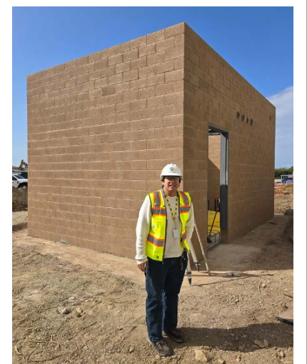
Tran visiting the active construction site at Malibu Middle School as part of Element Consulting's Summer Internship Program.
